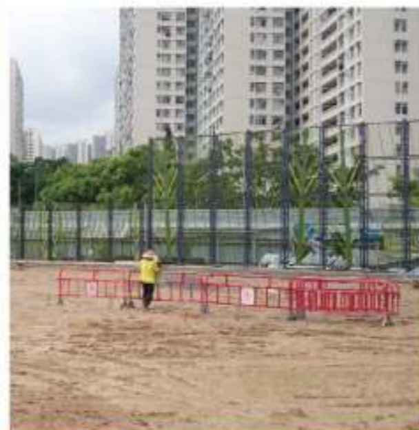
施工现场实拍 Construction site shooting 38-39
